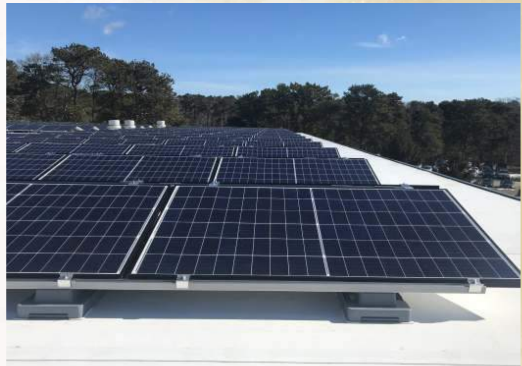
SOLAR PANEL INSTALLED ON ROOFTOP
